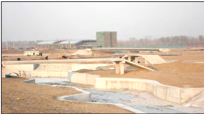
The Slalom course under construction
